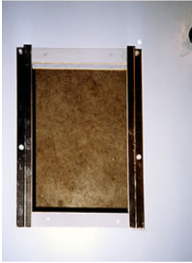
Install channel on inside of building Photo 1
