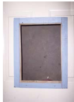
Installed door trim kit. Photo 6
