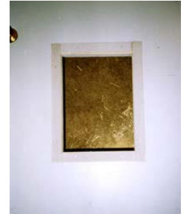
Frame the inside and outside of the hole on the door – use 3/8" cedar, pine or plywood strips – 1-3/4" or 2" wide. Photo 4
