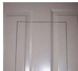
Draw template/drill 1/2" holes. Opening 12-1/2" x 17-1/2" on the Heavy Duty Dog Door®, 16-1/2" x 25-1/2" on the Big Dog Door™.
