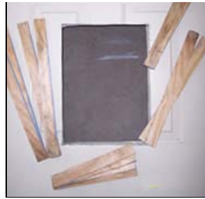
Cut raised panel door surface same as Photo 1 (Order Pet Door Trim Kit) Photo 2
