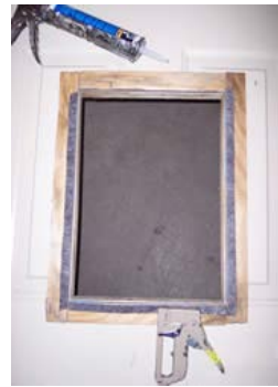
Use silicone caulking around trim kit for add insulation. To quiet door closing staple 5/8" window felt to sides and bottom. Photo 5
